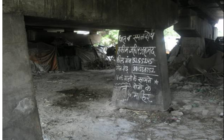
Figure 3: Unnatural and unhygienic flooring.
