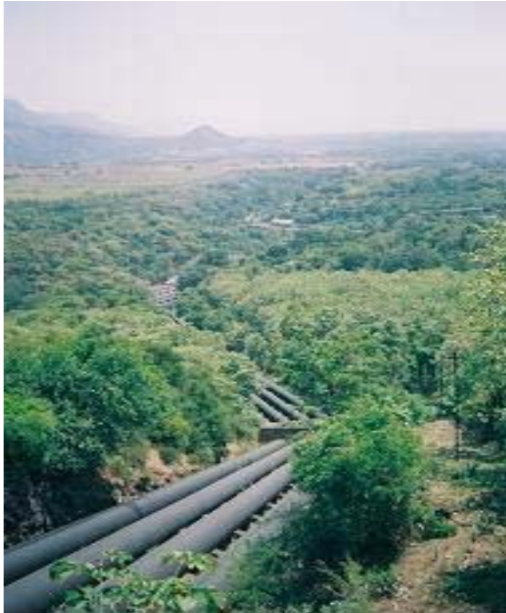
A view of Periyar Hydroelectric project at Lower camp, Gudalur
