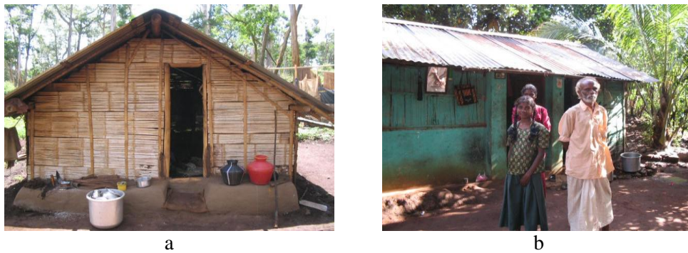
Figure 29a and b: Housing facility provided to mahouts in forest camps
