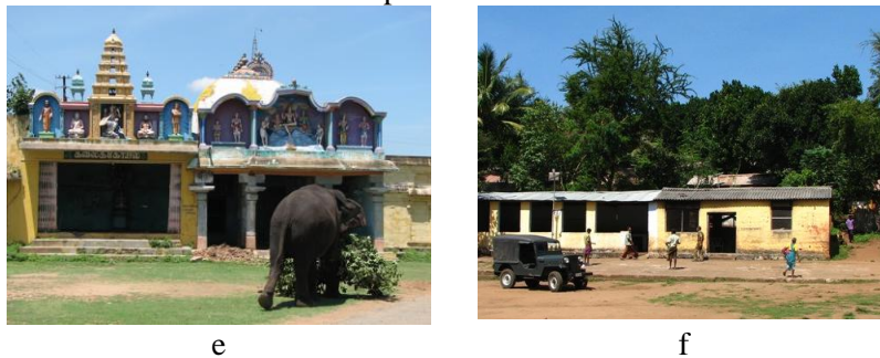
Figure 5e and f: Man-made shelters with roof made of concrete
